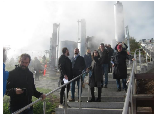
Image 29: People can walk/hike to the top of the ARC power plant and get a stunning view of surrounded area and the city of Copenhagen (Source: COWI)
