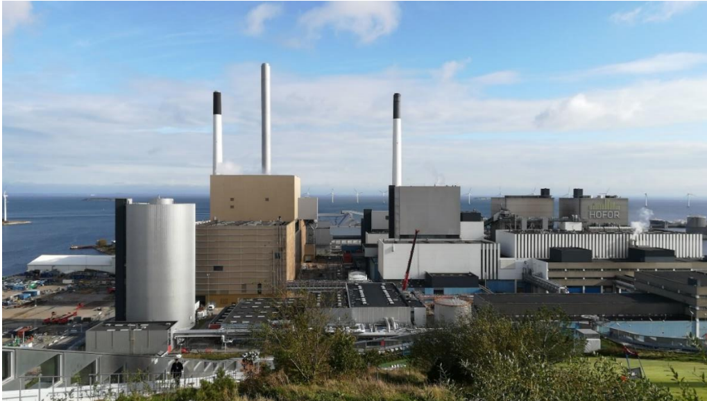
Image 30: BIO4 new woodchip-based cogeneration plant serving Copenhagen (Source: COWI)
