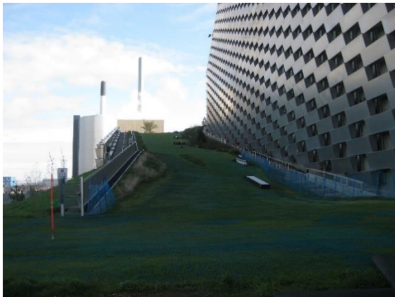
Image 28: View of the last part of the ski-slope placed on the ARC power plant (Source: COWI)
