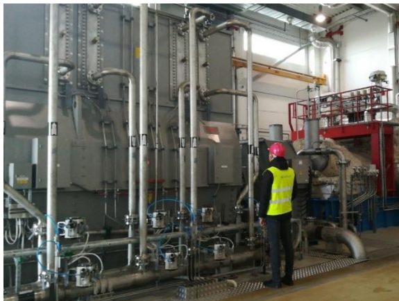
Image 20: Overview of the electricity production system at Örtofta power plant. From the left, it is possible to see the generator, the gear box and the turbine (Source: COWI)
