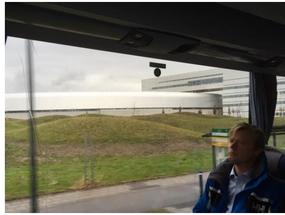
Image 23: MAX IV research facility in Brunnsög seen from the bus (Source: COWI)
