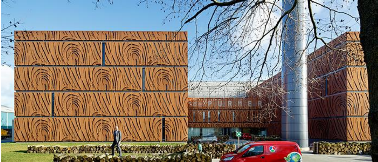
Figure 8: Biomass fired heating plant at Purmerend
